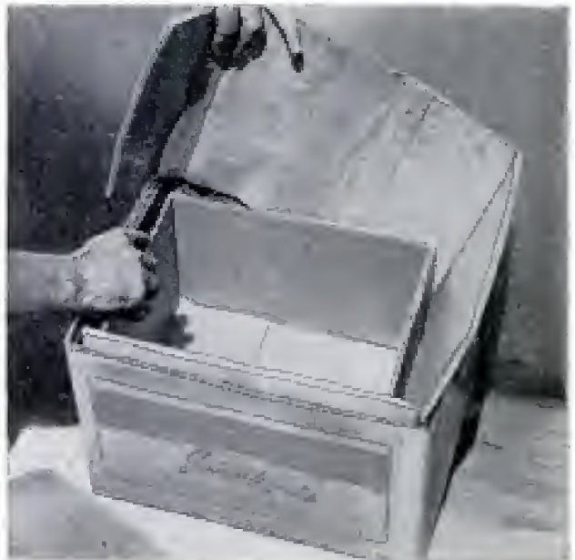
Cardboard from cut-up box is inserted between inner and outer cartons, above, to act as insulation
